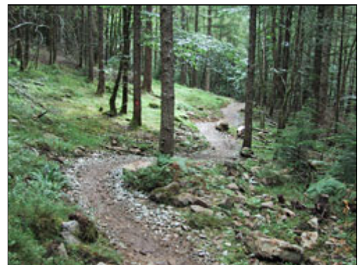
Create a rolling trail that dips and rises frequently. Click for bigger picture.
