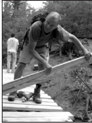
Bill Lindler building bridge
