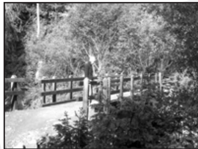
Last year's bridge work still standing
